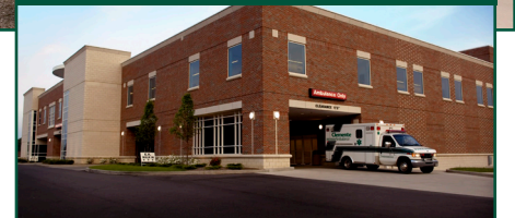
EMERGENCY ROOM ENTRANCE (REAR)
