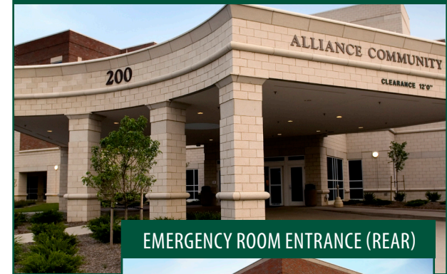
MAIN HOSPITAL ENTRANCE (FRONT OF HOSPITAL)
